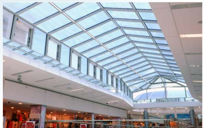
The Glass ceiling of Sahari Mall
